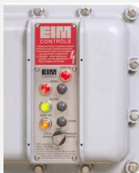
LOCAL/OFF/REMOTE 就地/停止/远程选择开关 OPEN/CLOSE/STOP 打开/关闭/停止按钮
